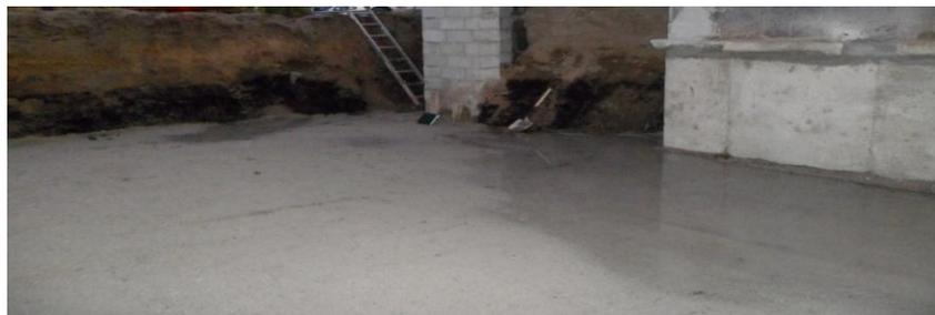
*Engineered fill ready for placement of footings.*
