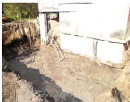
Every building rests on some kind of foundation whether it be footings and frost walls, piles, caissons or floating slab. Older houses were commonly built on rubble and mortar foundations. Considerable thought goes into the selection of a foundation design which depends upon soil conditions, local design factors and building use and should be done by an Engineer.
