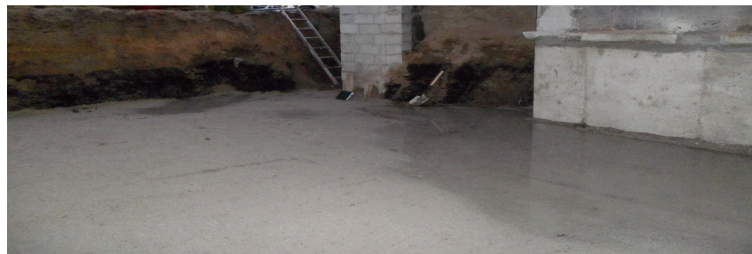
Engineered fill ready for placement of footings.
